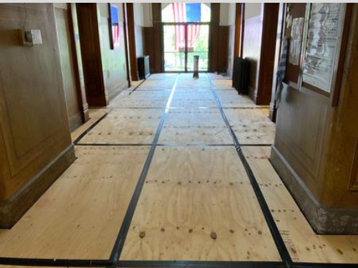
After Flooring Protection
