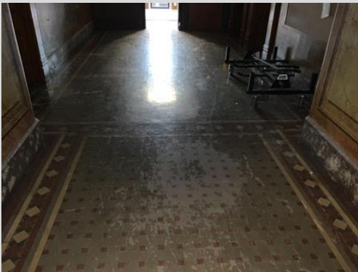
Before Flooring Protection
