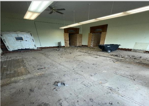
Flooring Demo 1 st Floor
