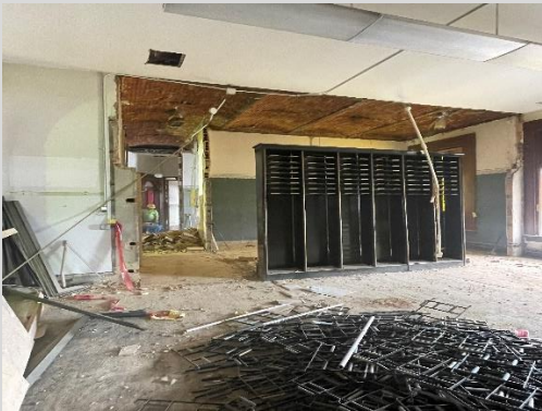
Wall Demo 2 nd Floor
