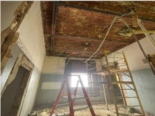
Ceiling Demo 2 nd Floor
