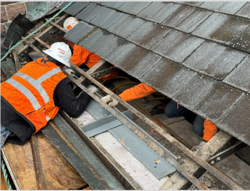
Installation Of North Elevation Steel From Exterior 1/31/24
