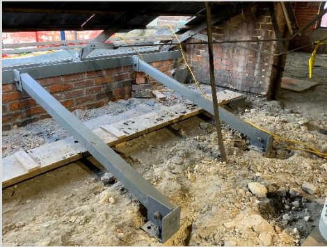
Steel Install Along The Inside of the North Attic Wall 2/2/24
