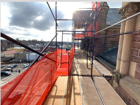
Top Level Of Scaffold Along the East Elevation 2/2/24
