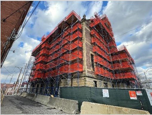
South & West Side Scaffolding 2/9/24
