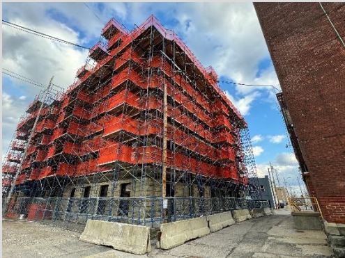
North & West Side Scaffolding 2/9/24
