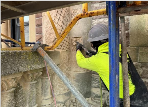
East Elevation Stone Patching Prep 3/1/24
