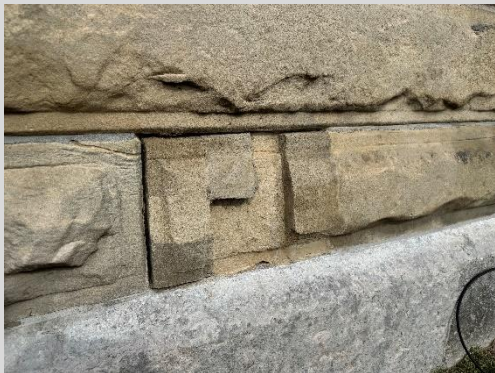
Stone Patching Mockup & Samples 3/1/24
