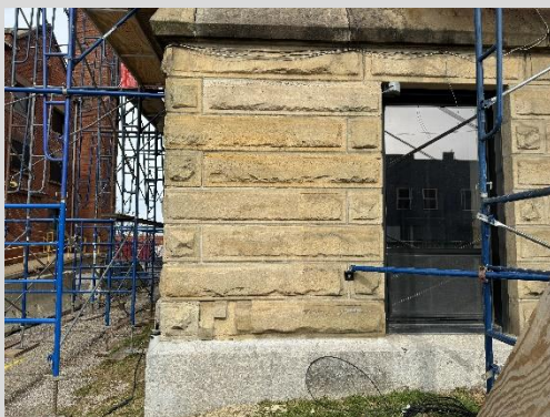
Stone Cleaning Mockup 3/1/24
